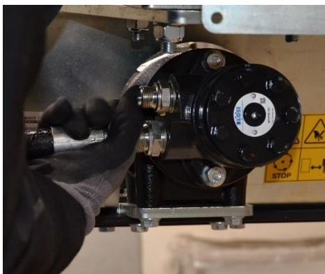
3 – 2 pcs. hydraulic hoses are mounted.
