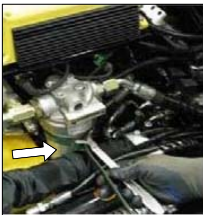
◀ Hydraulic oil filter location
